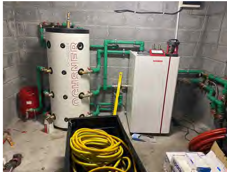
The heatpump installation in the plant room at the pilot site.
